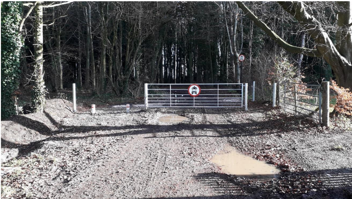
Typical Kent carriage gap (alongside gate) – Druids Lodge, installed October 2018 by Wiltshire Council
